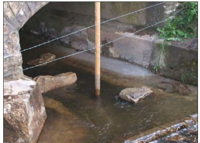
Large stone baffles held in position on concrete apron with stainless steel dowel rods drilled into both the apron and stones. (Poor placement of the livestock fencing as shown in the photograph has the potential to cause blockage by catching debris.)
